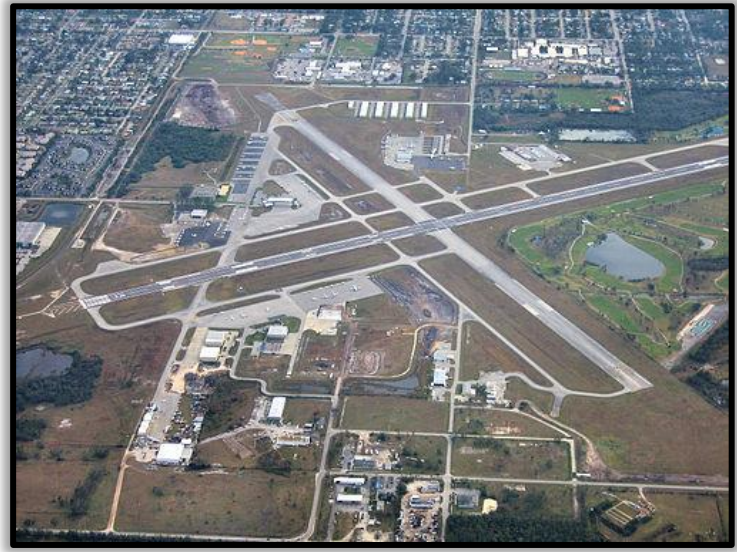
Figure 7 Kissimmee Gateway Airport
