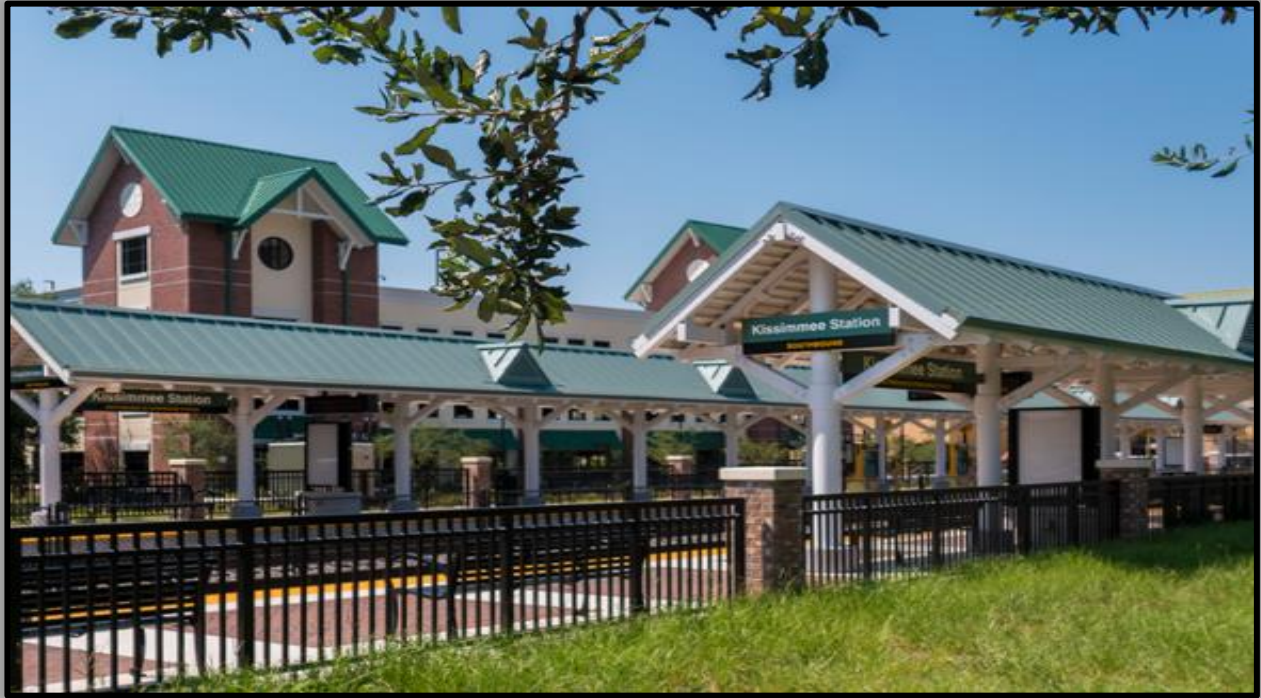
Kissimmee Intermodal Station, Courtesy of SunRail
