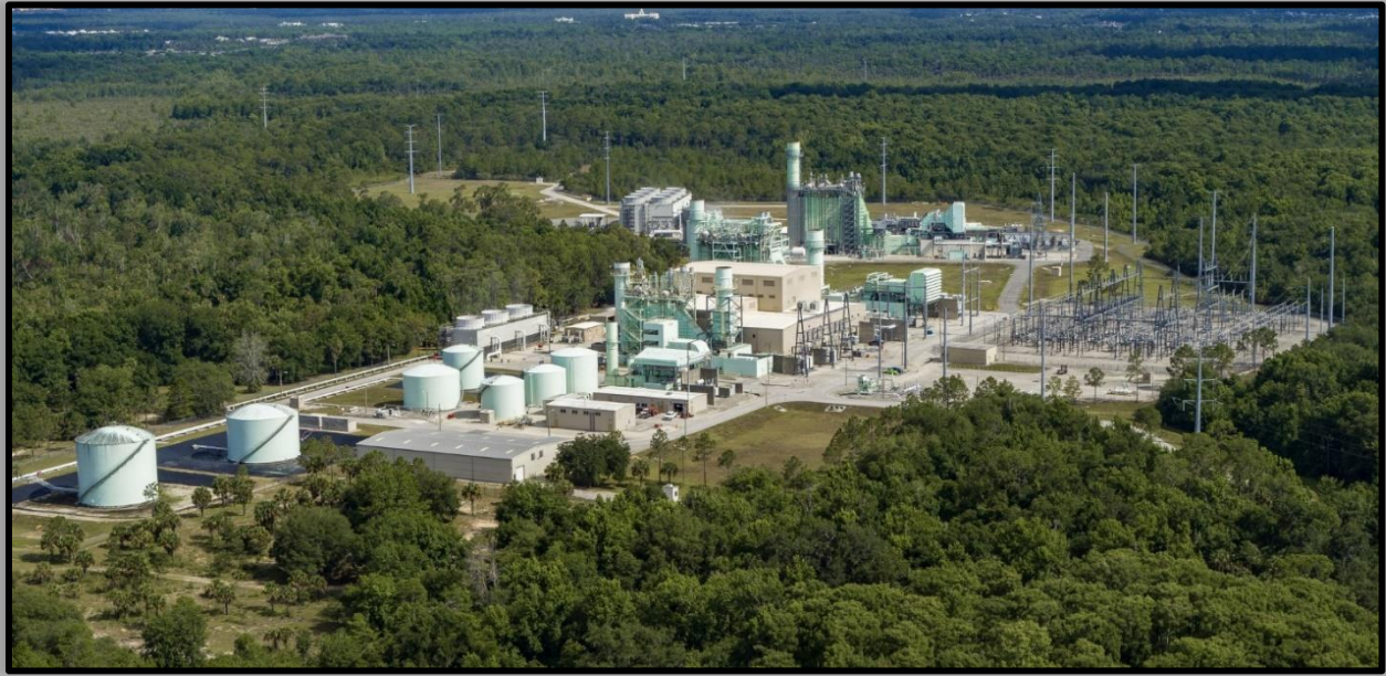
Figure 13 Cane Island Power Plant, Compliments of KUA
